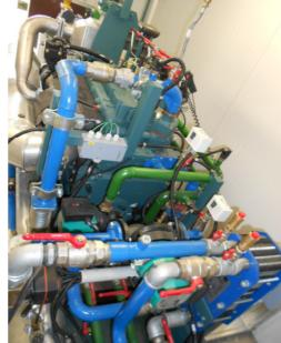
D. B-45 gasengine CHP House-scale Small Powerplant NRG MINI P50 SP NG type CHP unit A CHP unit Technical datas/specifications: CHP type: NRG MINI SP50 NG Motor type: NRG 50 G4LTi (Perkins 1004 G) 4 cycle, lined 4 cylinder motor with turbo charger Electric output: 50 kW, Thermic output: 66 kW, Total energy output: 116kW Generator: Mecc-Alte Eco 32-1L/4 0,4 kV, 50Hz Elecric efficiency: 34%, Thermic efficiency: 50%,
